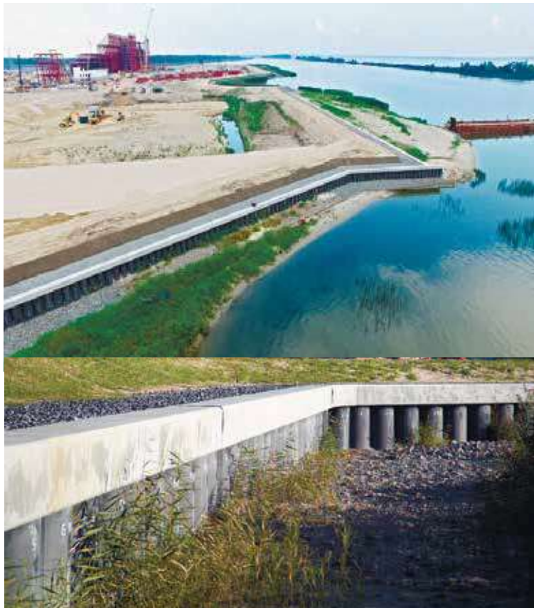
Construction of shore protection structures
